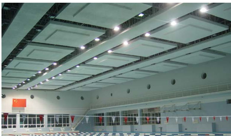
NATIONAL SWIMMING TEAM TRAINING CENTER - BEIJING, CHINA | SonaSpray "fc" White | 18,000 sf - 3/4" Thick
