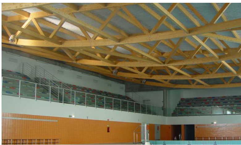
CAMPO DE OURIQUE MUNICIPAL POOL - LISBON, PORTUGAL | SonaSpray "fc" LIGHT GRAY | 1-1/4" Thick
