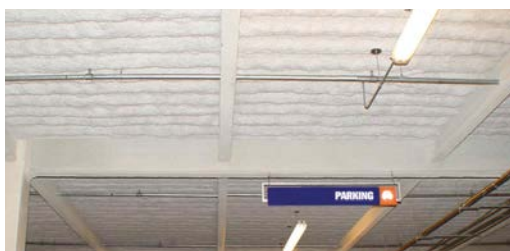
BASKETBALL HALL OF FAME - SPRINGVILLE, MASSACHUSETTS, USA K-13 Light Gray | 75,000 sf - 3" Thick
