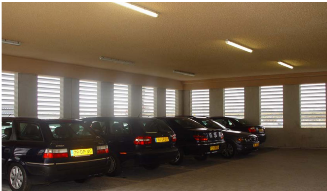
RESIDENTIAL COVERED PARKING - NIEUWEGEIN, UTRECHT, THE NETHERLANDS | SonaSpray "fc" Custom Color Beige | 4,800 sf - .50" Thick
