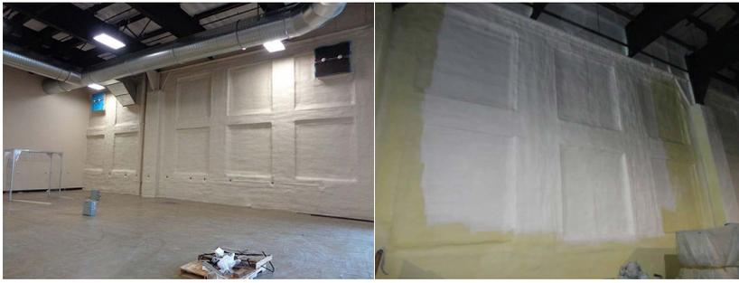
And when the R&A crew arrived on site, they could suit up and begin spraying. The surface prep work was performed by another company. "All the power washing, cleaning, and degreasing of the walls had already been done for us," says Anderson. "We could get right to work." First, they suited up in Tyveks with "the sprayers wearing 3M's full-face fresh air masks with canisters on belt packs," he continues.
